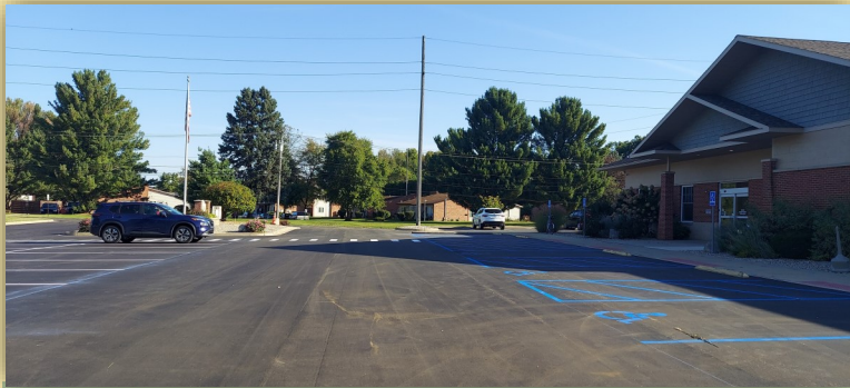
Picture of our newly rebuilt parking lot!
